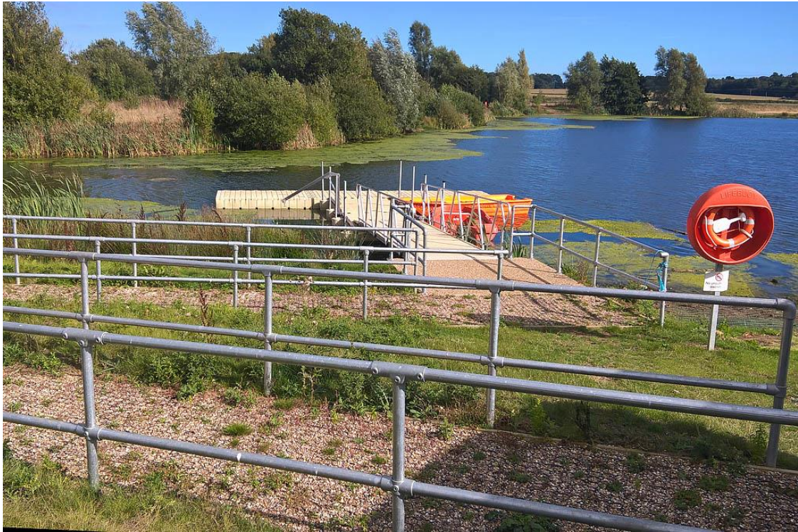
Photograph 1: Pontoon access point to the lake.
